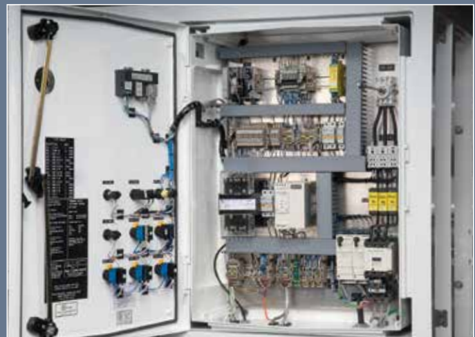
Interior door / electrical
